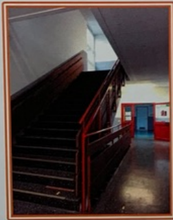
This is the staircase in the building A.
