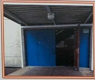
This is the entrance on the building A.
